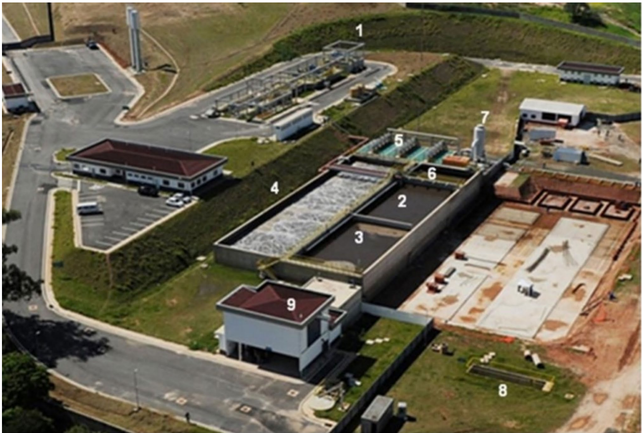
Fig. 1 Aerial view of the Water Resource Recovery Facility (WRRF). Units: (1) preliminary treatment, (2) anaerobic tank, (3) anoxic tank, (4) aeration tank, (5) membrane tank, (6) deoxygenation tank, (7) treated effluent tank, (8) Parshall flume, and (9) sludge dewatering building
