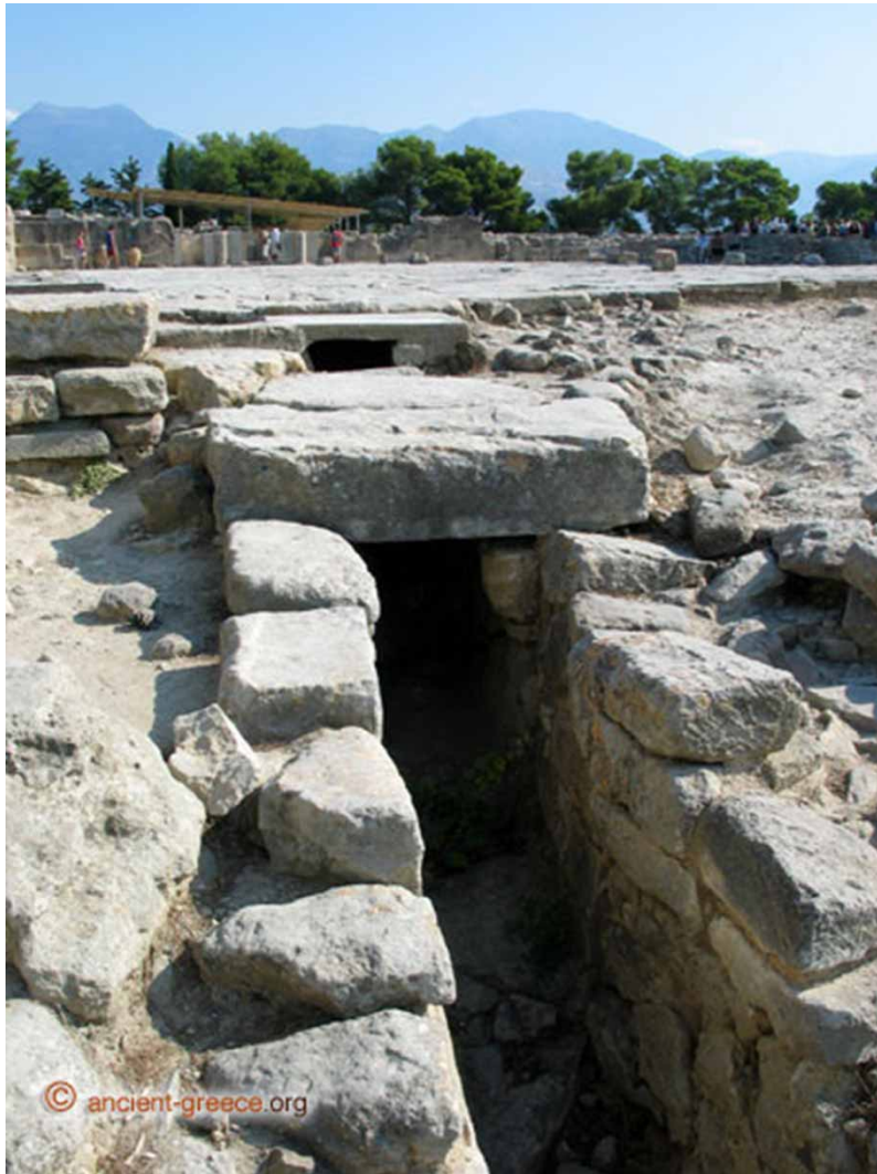
Fig. 3 | Tunnel for transporting wastewater in the Festos palace to agricultural land. Source: Angelakis et al. (2018).
