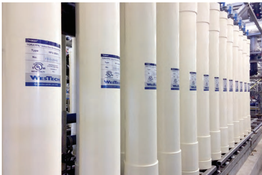
Figure 1: UF/RO system designed and constructed by WesTech Engineering
