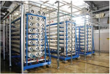
Full-scale UF (VersaFilter™) and RO systems built by WesTech Engineering, Inc. (photo credit WesTech. <a href="www.westech-inc.com">www.westech-inc.com</a>).
