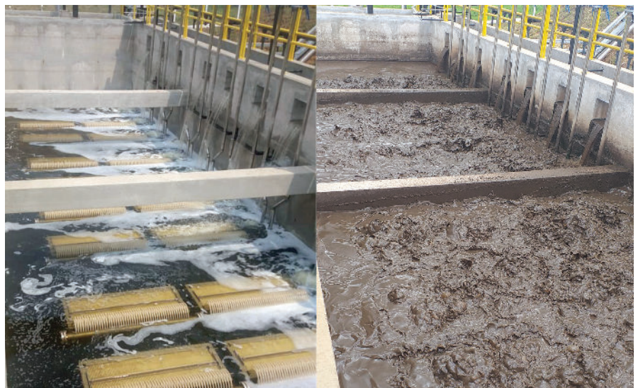
Figure 1(top): one train MBR tank containing 10 Toray MBR modules
