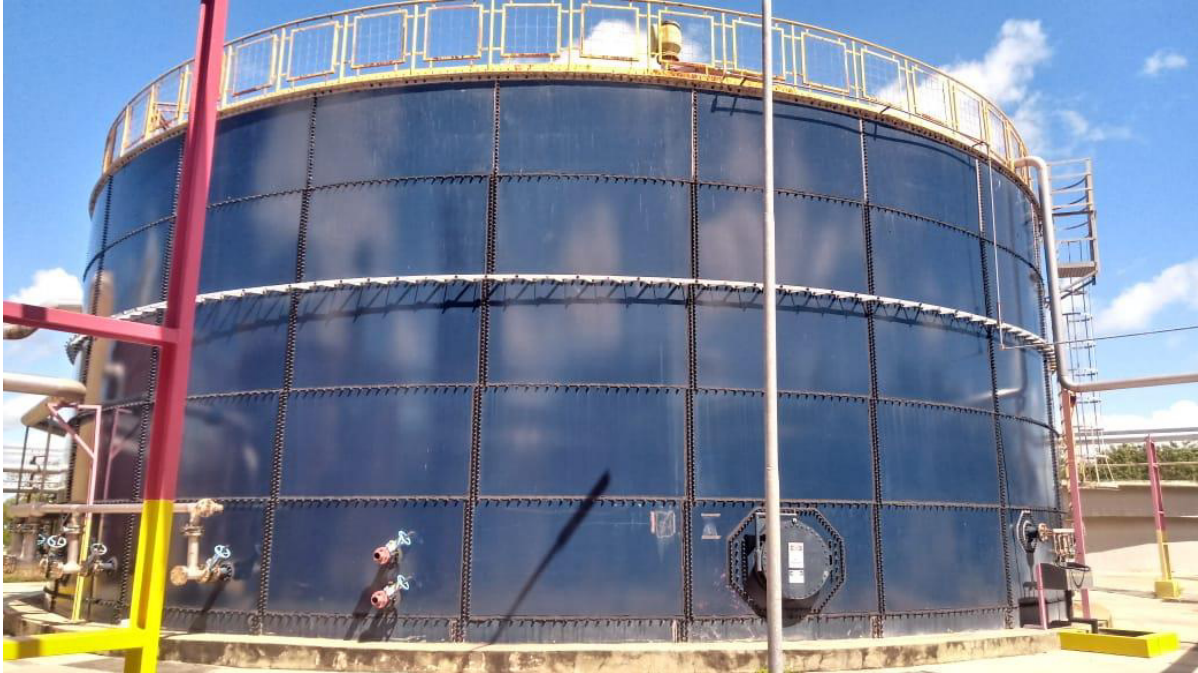
Figura 21 – UASB ( Upflow Anaerobic Sludge Blanket ).
