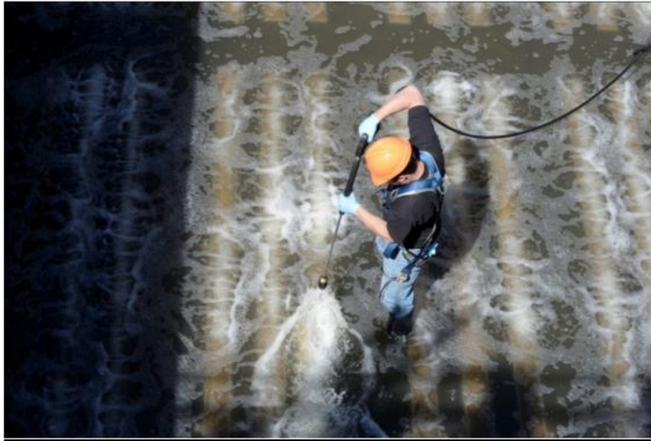
Figure 5. A worker pressure washing the 12-year old diffusers in the north tank in 2013. It took 3-4 hours to pressure wash the entire tank.
