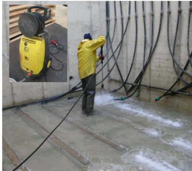
Figure 4. Pressure washing the eleven-year old diffusers at the factory test tank in 2012. The positive effects of pressure washing can be seen on the air distribution pattern.
