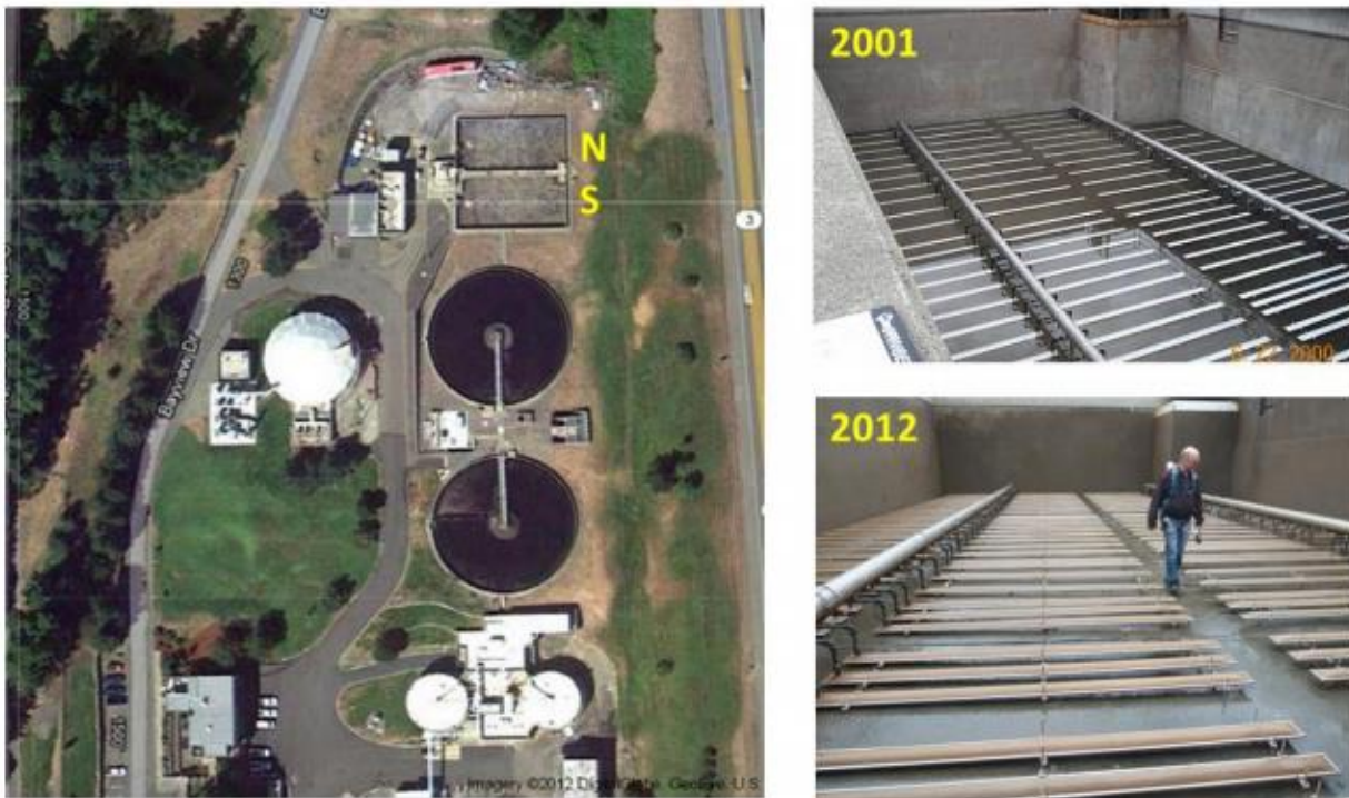
Figure 1. Bremerton Plant. Left photo shows the two basins. Top right photo shows the north basin shortly after installation and the bottom right photo shows the north basin immediately following the 2012 off gas testing.
