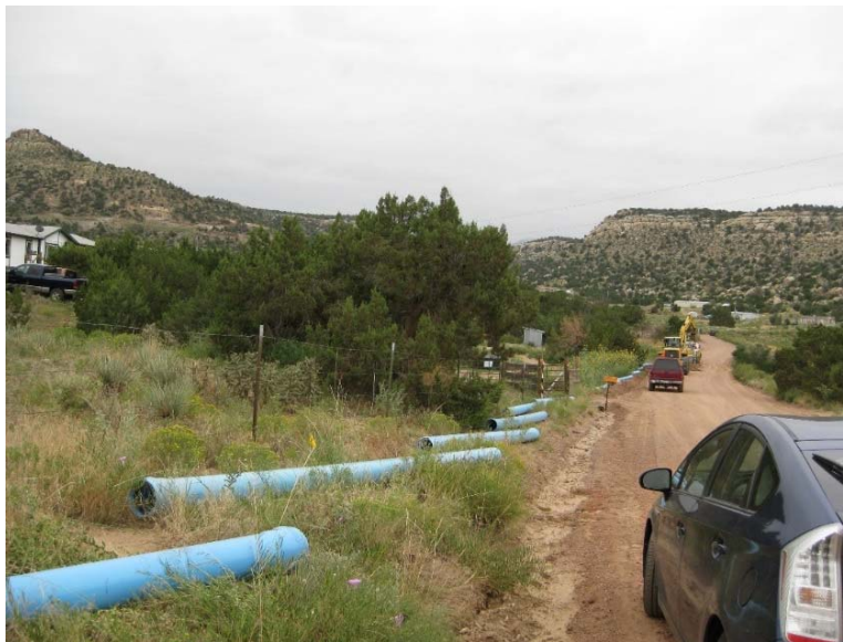
Figure 1.1 Installation of new PVC distribution piping in Williamsburg, Colorado
