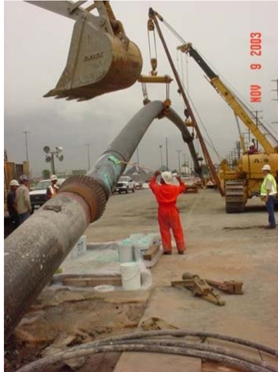
Figure 4.1 LADWP HDPE pipe installation by HDD in Los Angeles Harbor
