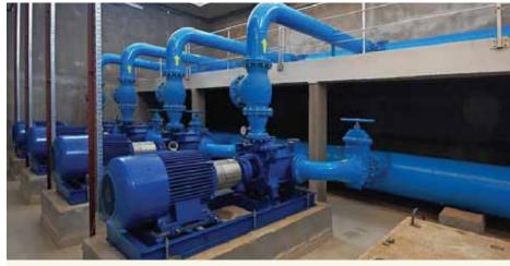
Image 16: A major pump station in a water distribution system. (Source: DMU, 2015)
